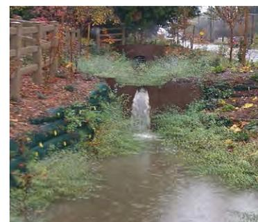
A stair-stepped pool slows runoff in Seattle's NW 110<sup>th</sup> Cascade project.
