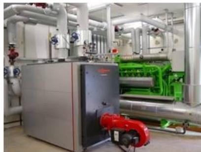
***Heat only biogas boiler***
