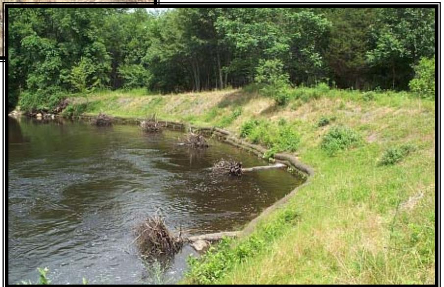
**Restoration of streambank and growth of vegetation one year after project completion.**
