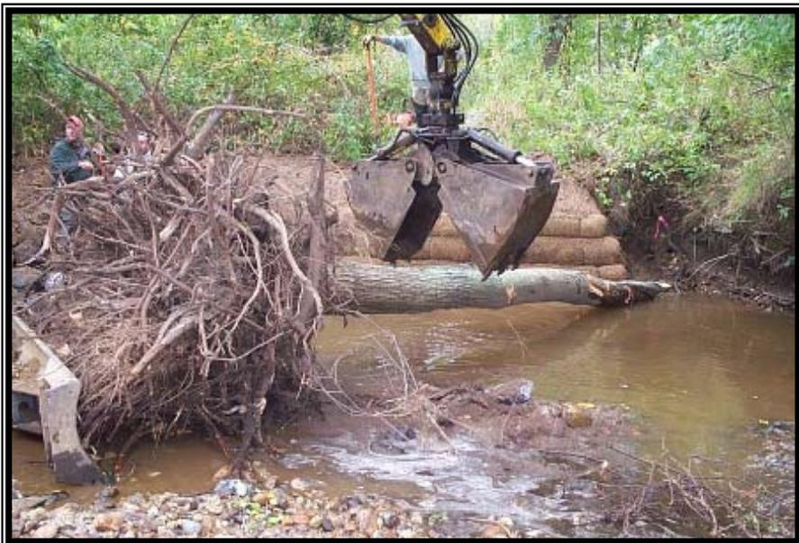
**Installation of tree and rootwad to deflect flow away from bank, provide for overhead fish habitat, and scour instream habitat.**
