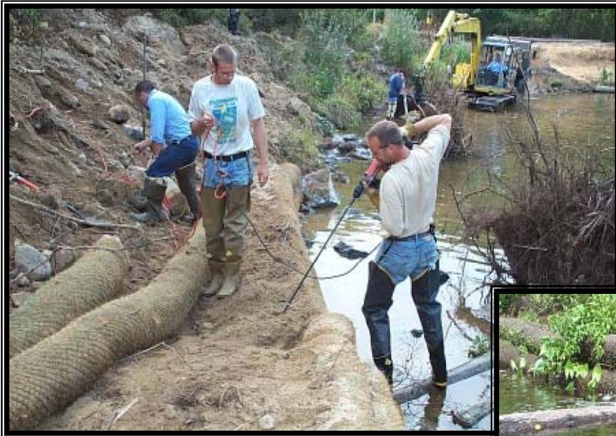
**Installation of triple layer coir fascine to stabilize toe of slope.**
