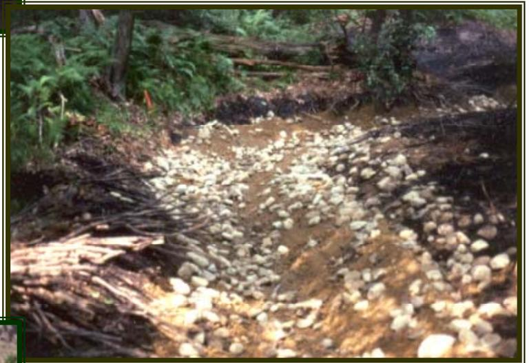
**View of new channel relocated into wetlands immediately post restoration.**
