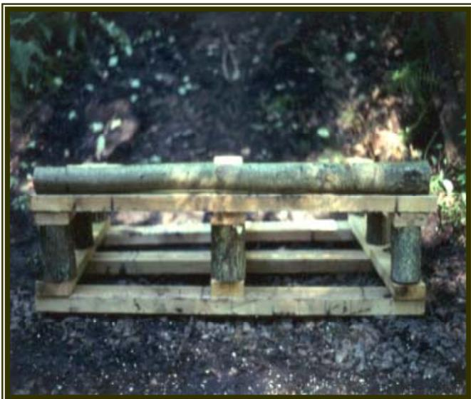
**Prefabricated LUNKER constructed of oak planks prior to installation.**
