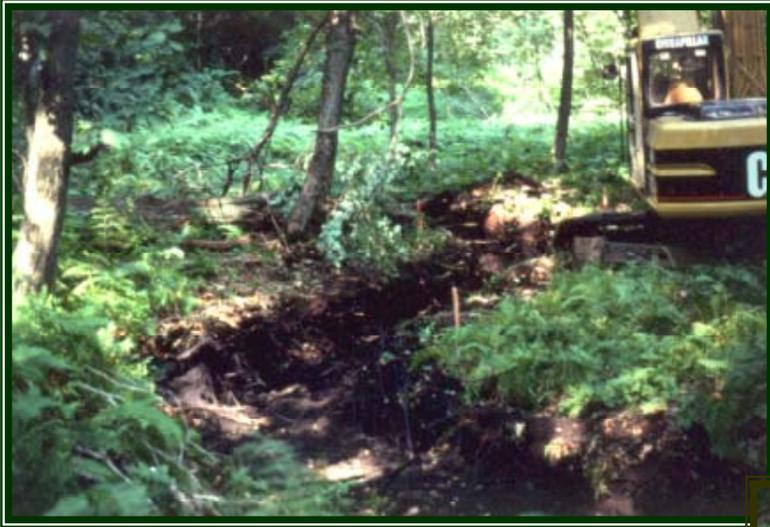
**Rough-out excavation of new channel being relocated into wetlands.**
