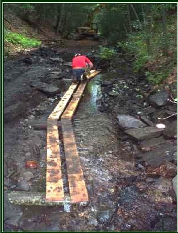
**Installation of modified LUNKER, a fish habitat enhancement structure designed to create undercut bank habitats.**
