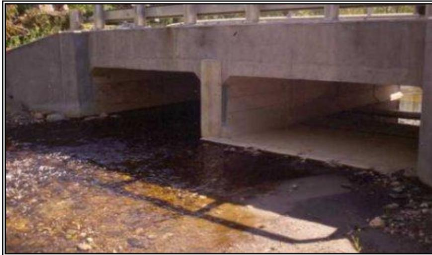
Figure 7. Culvert on left is sunken 1 foot below grade. Culvert at right, installed “at grade” accommodates high stream flows.
