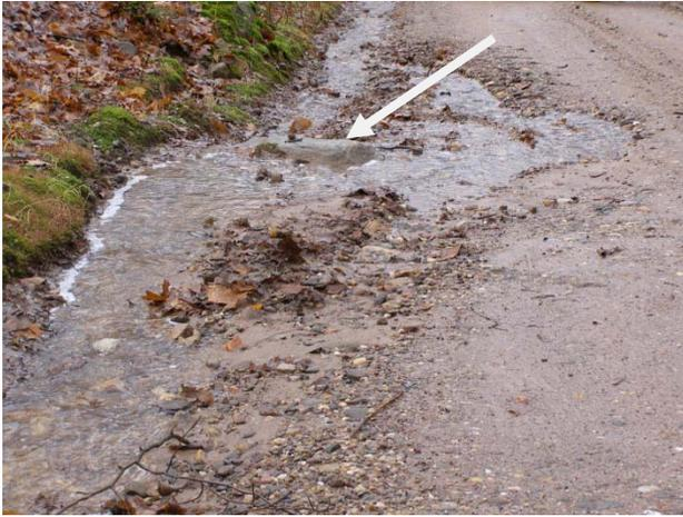
Recommendations set forth in the Connecticut Best Management Practices (BMP) guide section on Stream Crossings, state that “the top of the culvert should be covered with fill to a depth of at least one foot, or half the culvert’s diameter, whichever is greater, to protect the culvert from being crushed by vehicles.”<sup>5</sup>
