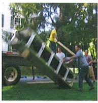
In the photos above, a couple of HVA staff members unload the Alaskan Steeppass units we'll be using for the Furnace Brook Fishway restoration project. Each of these units weighs about 450 lbs! The Steeppass units will be installed inside the existing fishway, creating an extremely durable baffling system that will maintain velocities that fish can handle as they move upstream.
