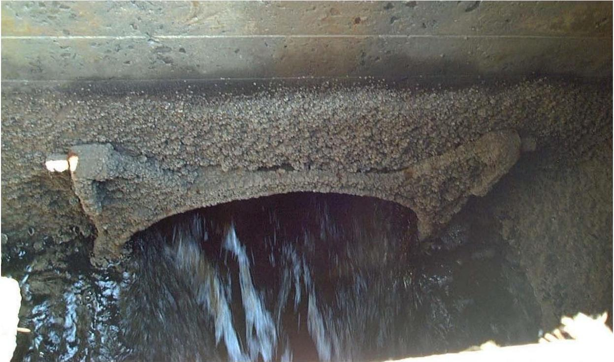
Water rushing out of upstream pipe and into tide gate chamber (after round metal tide gate had broken off)
