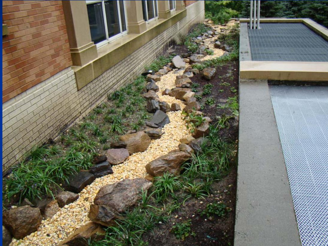
Mitigation of Stormwater runoff into grid area
