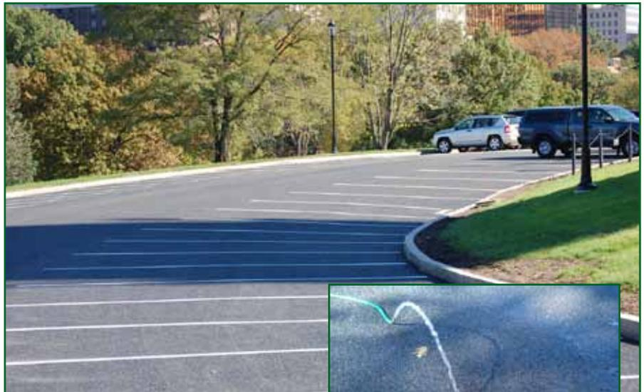
**Porous asphalt at the State Capitol parking area. Right: Demonstration of absorption capacity.**
