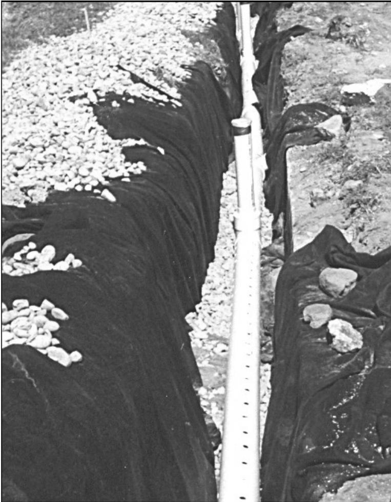
Figure 6.3. Installed underdrain pipe
