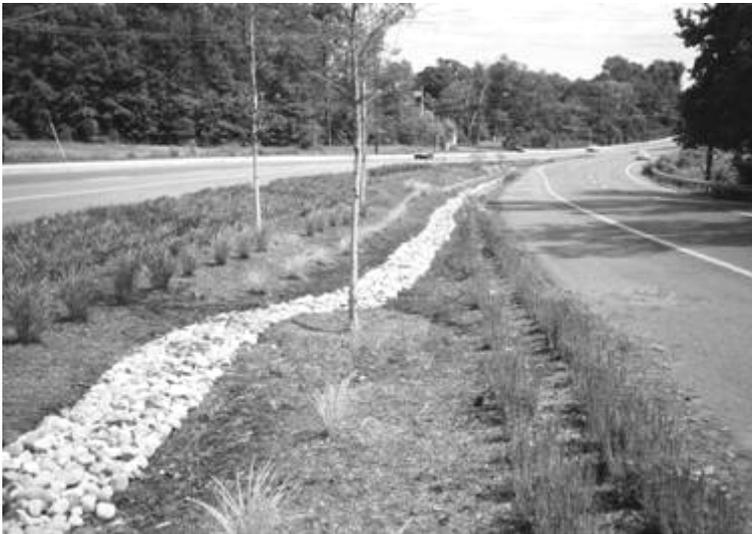
Figure 2.4. Median bioretention
