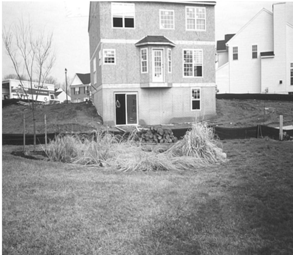
**Figure 6.1.** Silt fence around bioretention
