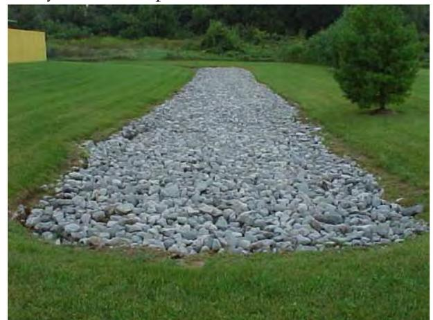
Figure 6.4.30 – Infiltration trench.
