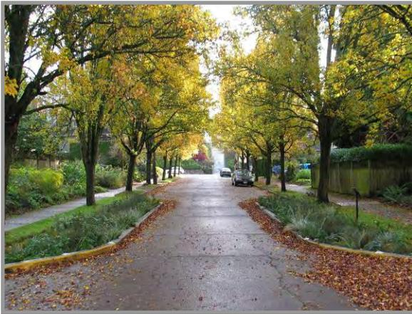
**Curbs are extended into street to construct bioretention areas and calm traffic.**
