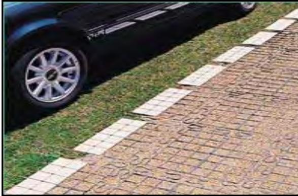
Figure 6.4.17 – Permeable pavement. Source: Adapted from Connecticut, 2004.
