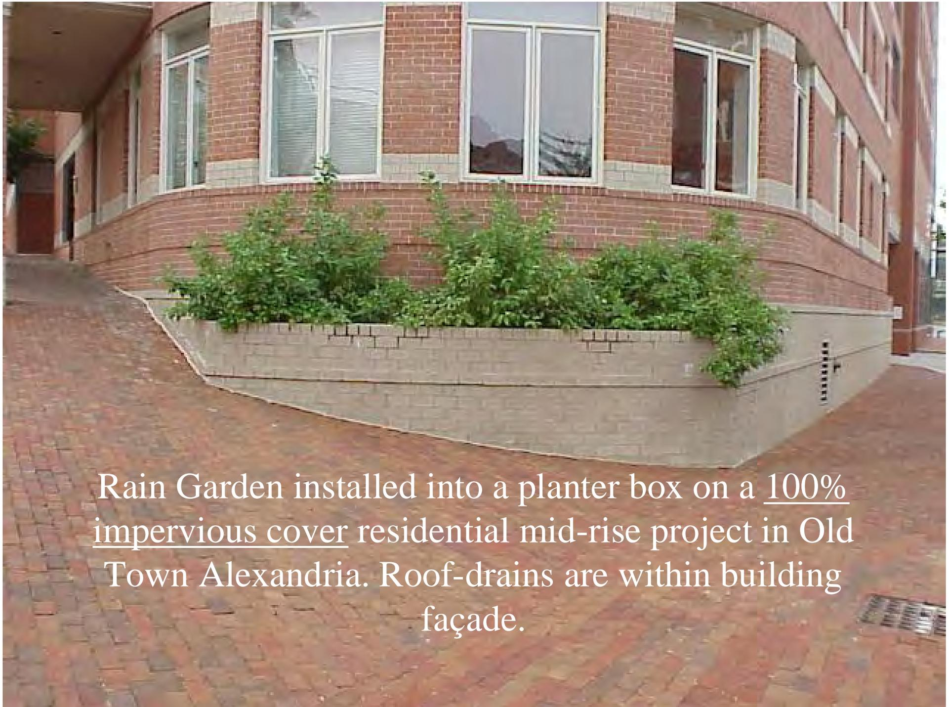
Rain Garden installed into a planter box on a 100% impervious cover residential mid-rise project in Old Town Alexandria. Roof-drains are within building façade.
