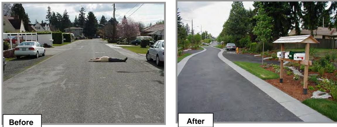
Figure 6.3.16 – LID urban retrofit project in Seattle, WA, using rain gardens/detention cells.
