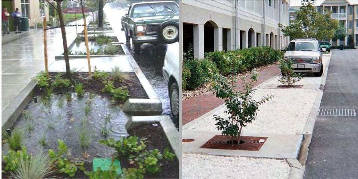
Figure 6.3.10 – Examples of planter box designs in high density development.
