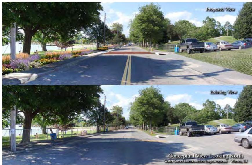
Figure 6.3.11 – Rain Gardens, Porous Paving Infiltration Chambers in a thickly settled Historic neighborhood and water front park.
