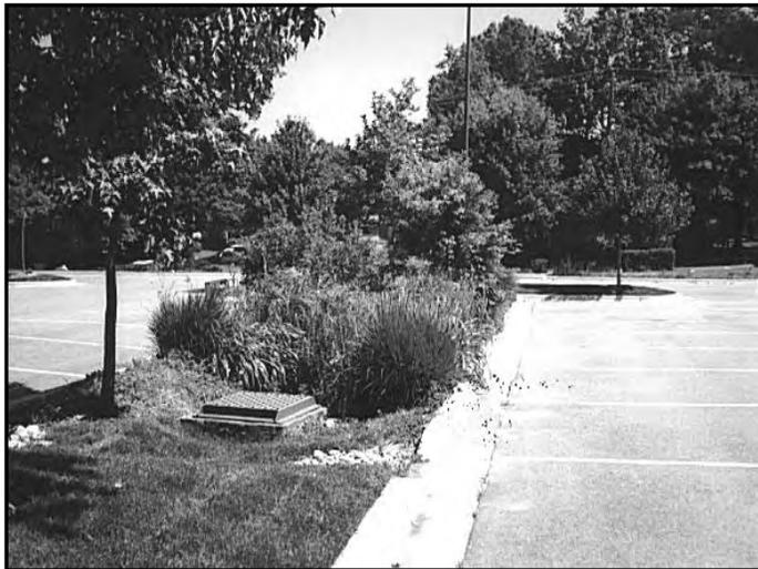
Figure 6.4.28 – Bioretention in use as a parking lot island.
