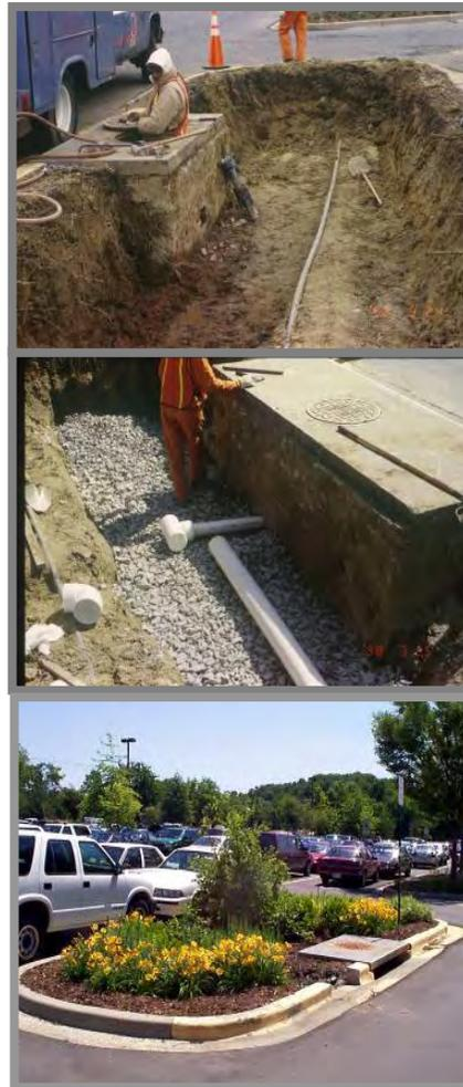
Figure 6.3.13 – Bioretention retrofit.
