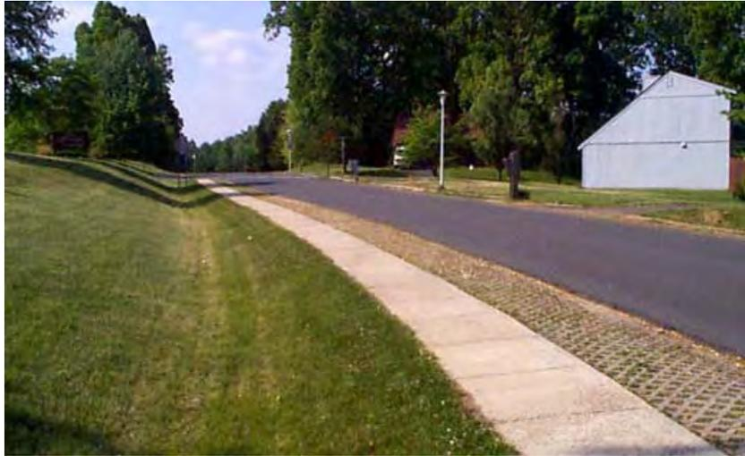
Figure 6.3.5 - Narrow road section with sidewalks, shallow swale and porous pavement shoulders.
