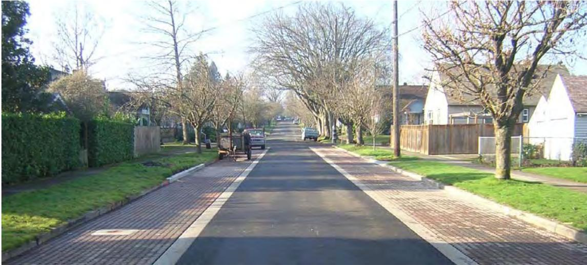
Figure 6.3.12 – Porous surfaces.
