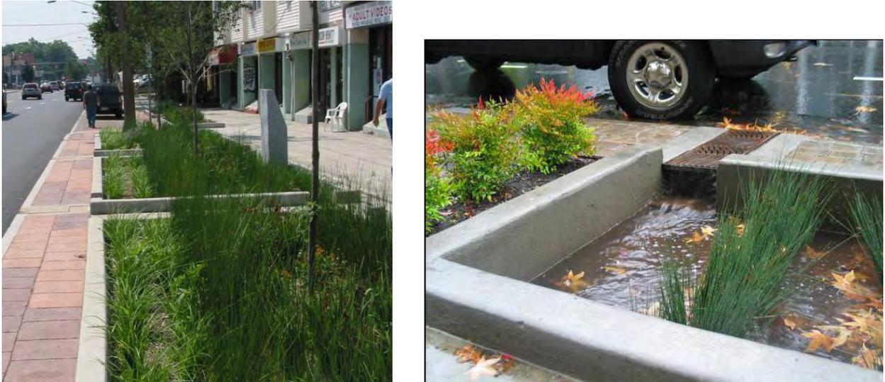
Figure 6.3.18 – Bioretention planters in Bridgeport, CT.
