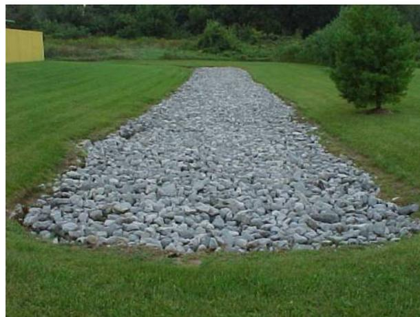
Figure 4.28 – Infiltration trench. Source: Connecticut Department of Environmental Protection.
