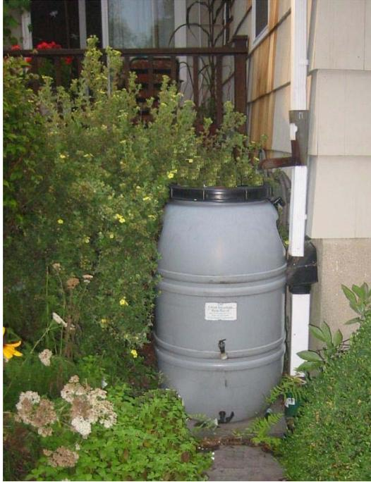
Figure 4.24 – Example of a rain barrel. Source: Connecticut Department of Environmental Protection.
