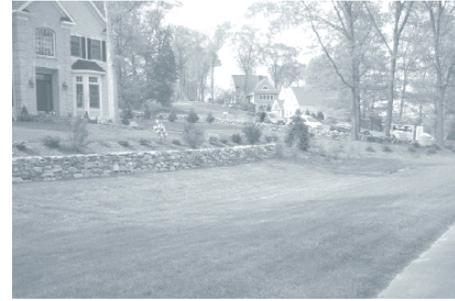
Figure 4.18 – Vegetative filter strip. Source: Connecticut, 2004.
