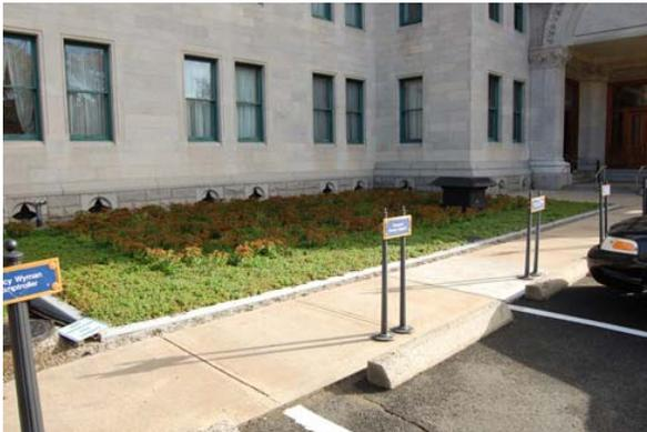
Figure 3.13 – Bioretention retrofit.
