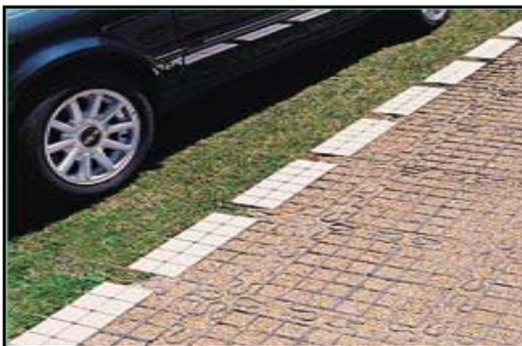
Figure 5.17 – Permeable pavement. Source: Adapted from Connecticut, 2004.
