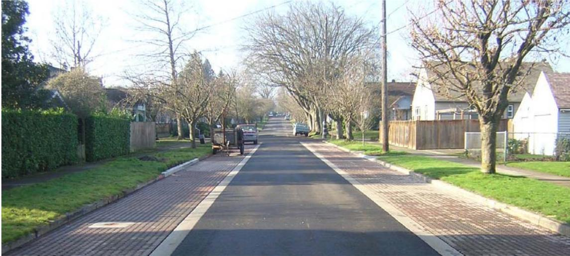
Figure 4.13 – Porous surfaces.
