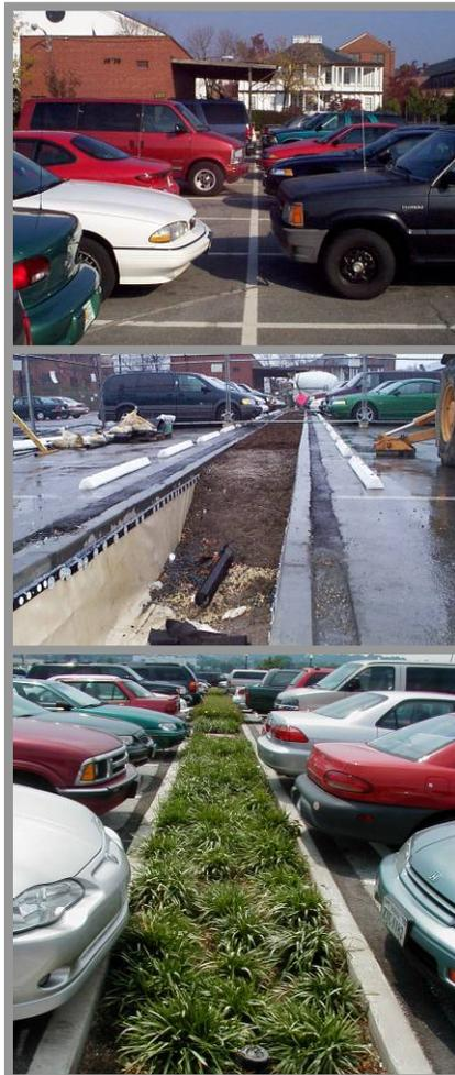
Figure 4.15 – Bioretention retrofit at the U.S. Navy Yard in Washington, D.C.
