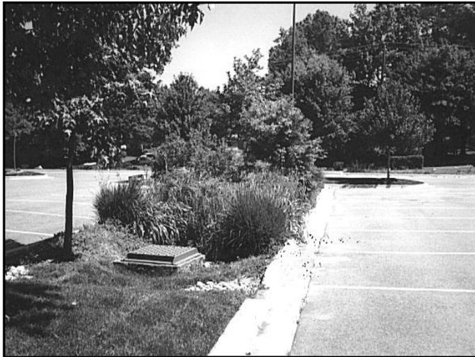
Figure 5.30 – Bioretention in use as a parking lot island.
