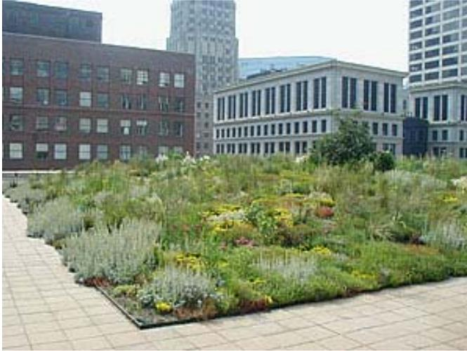
Figure 5.23 –Chicago City Hall green roof. Source: Photo (c) 2004 Roofscapes, Inc. Used by permission; all rights reserved.
