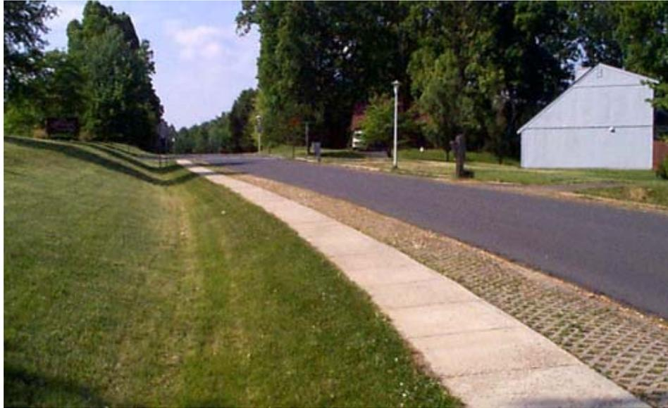
Figure 4.5 - Narrow road section with sidewalks, shallow swale and porous pavement shoulders.
