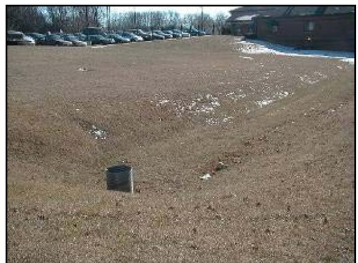
Figure 5.30 – Infiltration trench near a parking lot.
