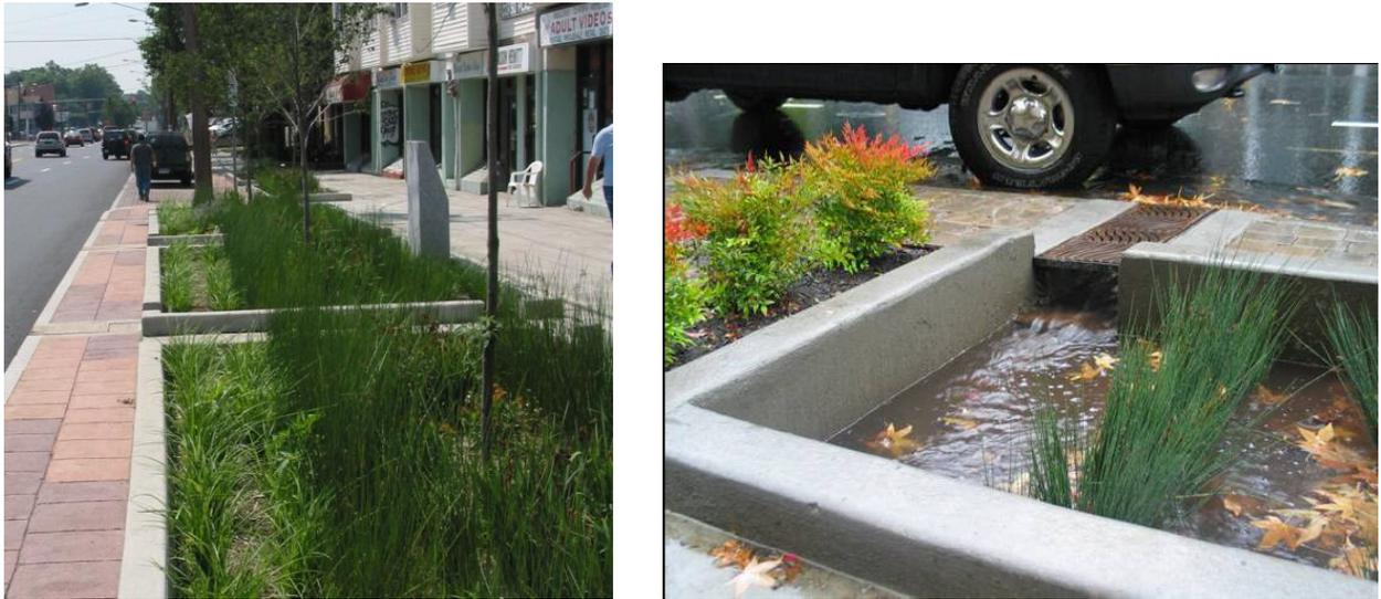
Figure 4.18 – Bioretention planters in Bridgeport, CT.
