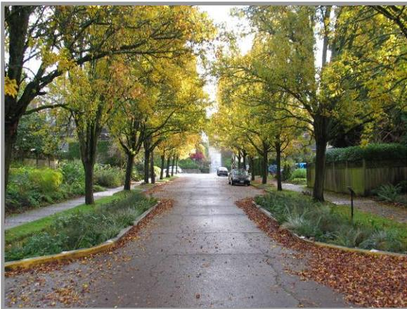
**Curbs are extended into street to construct bioretention areas and calm traffic.**
