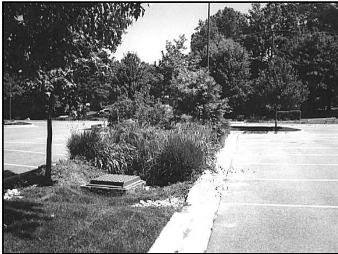
Figure 5.28 – Bioretention in use as a parking lot island.
