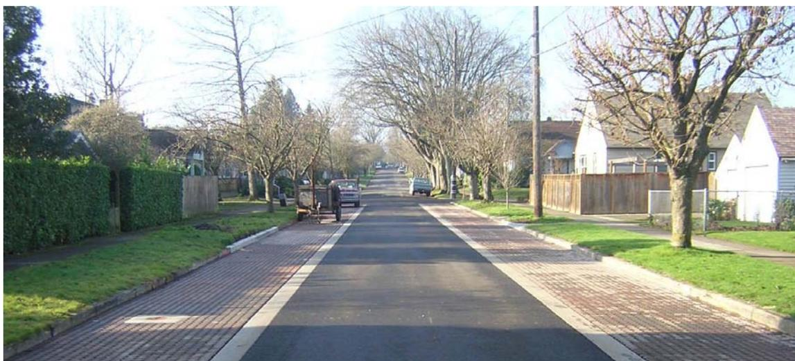
Figure 4.12 – Porous surfaces.
