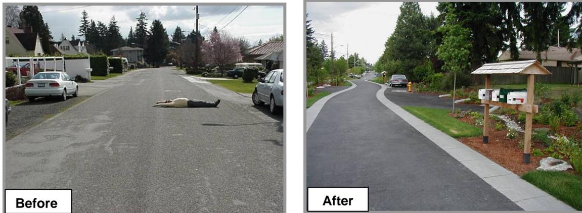
Figure 4.16 – LID urban retrofit project in Seattle, WA, using rain gardens/detention cells.
