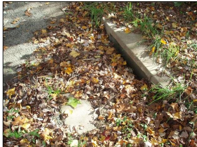
**Fig. 8-6. Storm drain on Lakeview Drive completely filled with sand and debris.**
