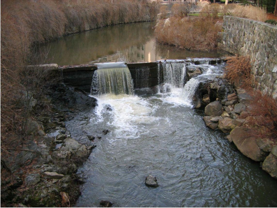
**Figure 4. An example of both a fish barrier (dam) and a modified channel in the Byram River.**
