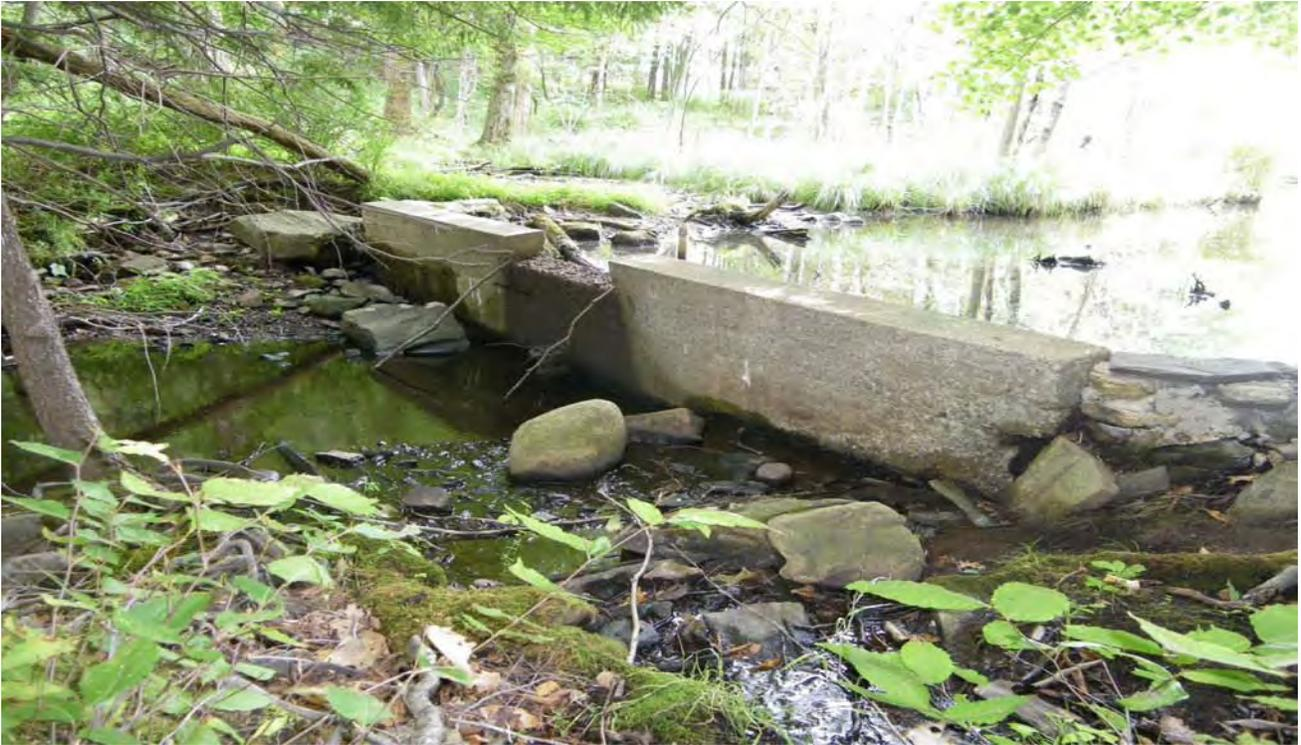
Typical Fish Barrier in a Headwater Stream of the Byram River Watershed.
