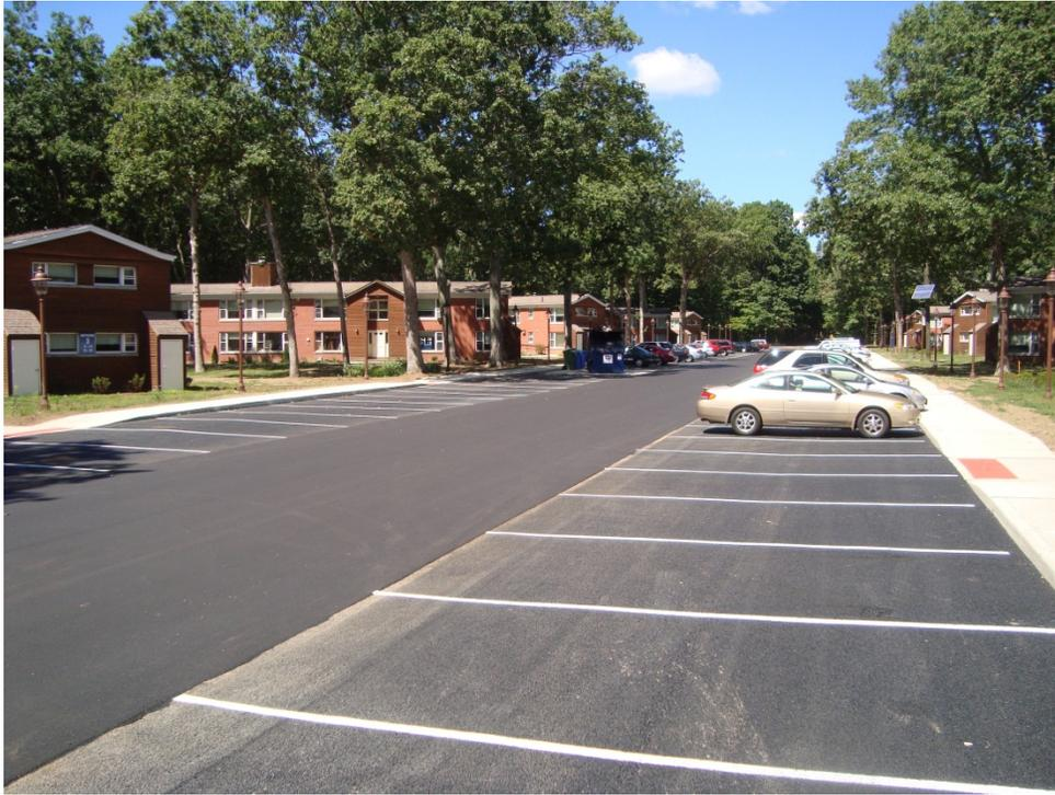
**Figure 12. Pervious asphalt at Northwoods apartments.**
