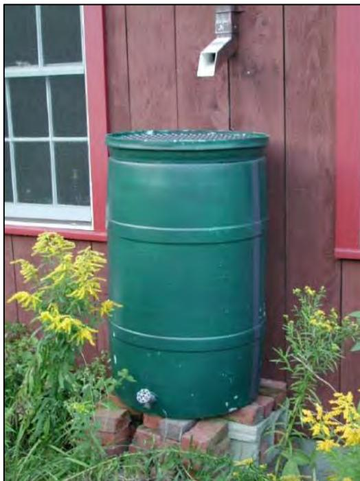
Figure 8-4. Example of a residential rain barrel.
