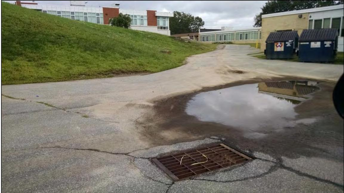
Figure 8-41. Deposition of eroded sediment near a catch basin at the school delivery area.
