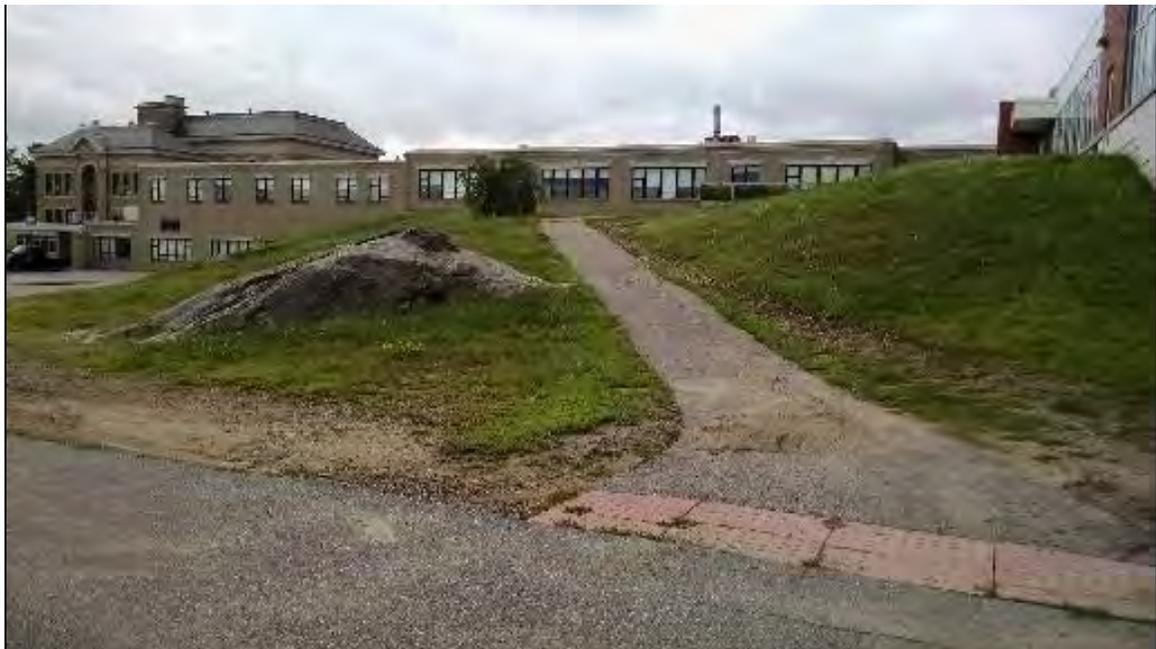
Figure 8-39. Erosion along a walkway and sediment deposition near the school delivery area.
