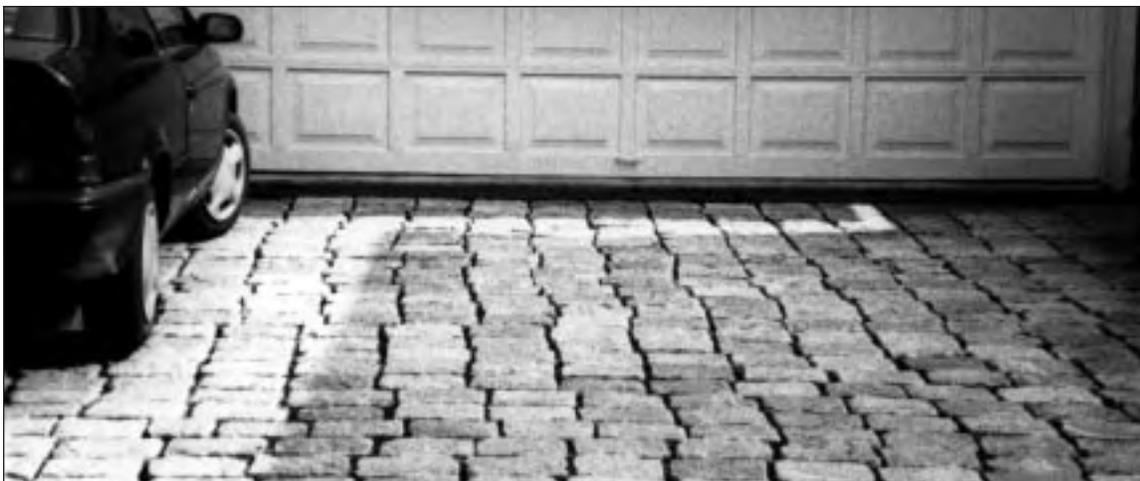
Using porous pavement, like this stone driveway, instead of impervious surfaces like blacktop increases infiltration and decreases runoff pollution.
