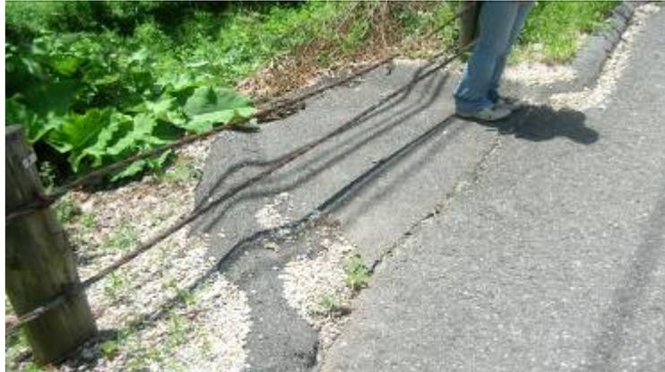
Curb Cut in Route 128 to Divert Stormwater Runoff Away from Travel Lanes
