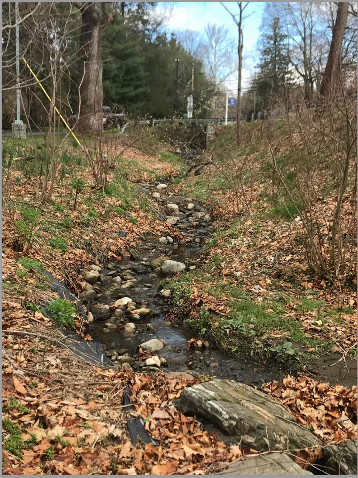
**Figure 5.27: Candidate site for step bioretention system to manage stormwater conveyance and improve channel stability; geotextiles from previous stabilization exposed**
