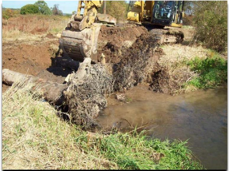
**Figure 5.17: Rootwad Placement. Source: Princeton Hydro**
