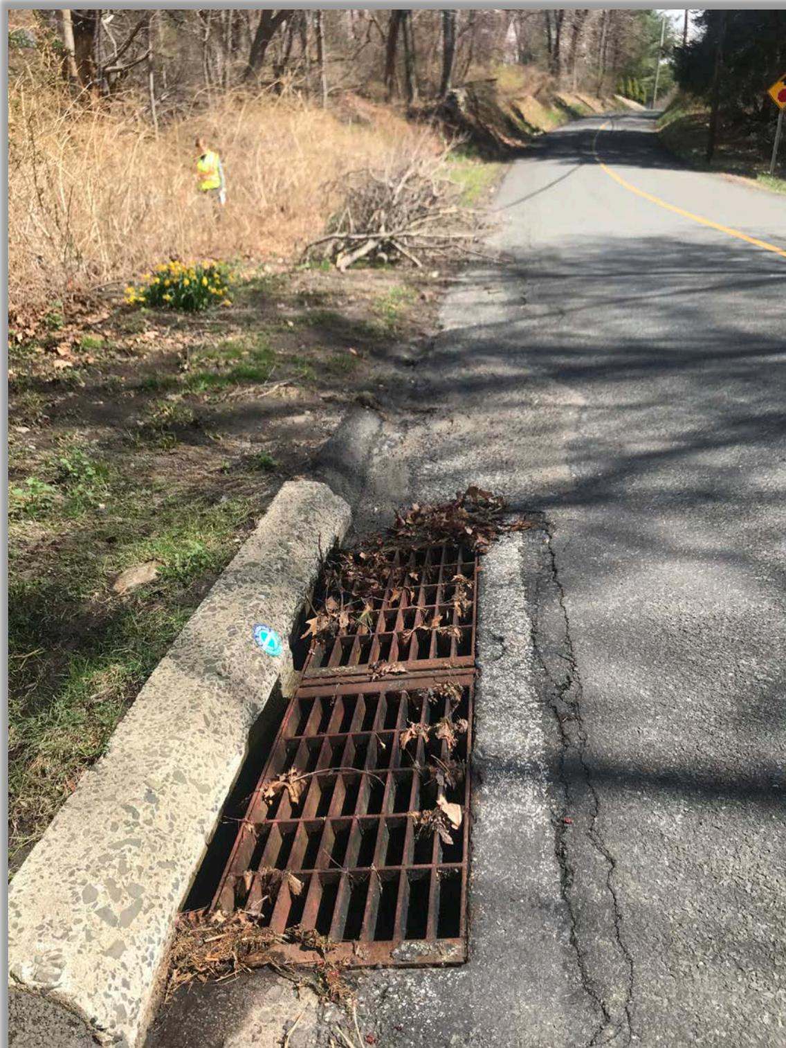
Figure 5.47: Beer Road catch basin to be retrofitted with basin insert
