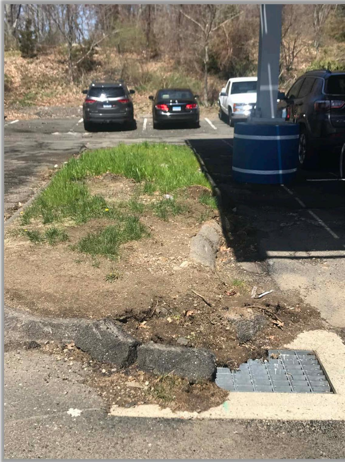
Figure 5.42: Parking lot catch basin inundated with eroding soils
