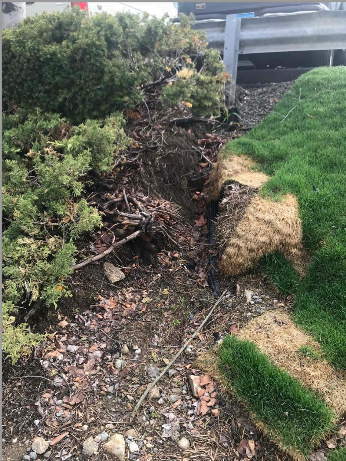
Figure 5.37: Parking lot runoff not adequately intercepted, leading to erosion
