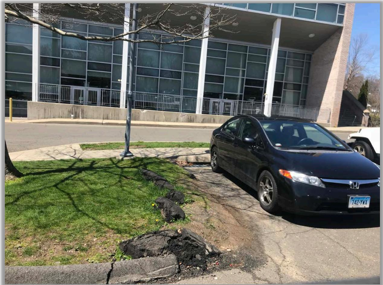
Figure 5.43: Another catch basin showing capture of leaf litter and solids from eroding lawn surface and poor state of repair for curbing
