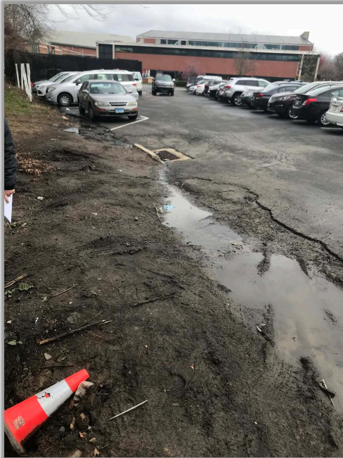
Figure 5.38: Poor stormwater management leads to ponding and generation of solids
