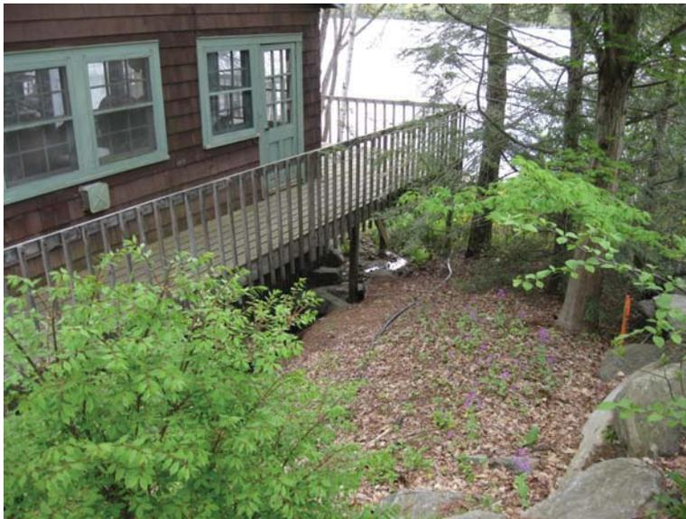
Drainage goes under existing deck & is flooding yard
