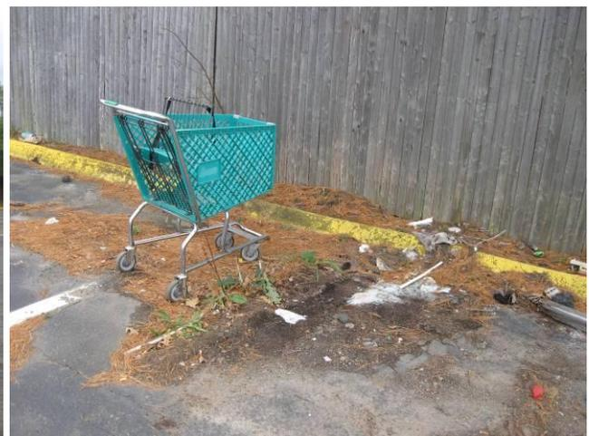
The parking lot pavement is breaking up and stained and sediment and debris have collected in some areas.
