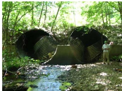
In addition there is a misaligned crossing under State Route 254. If this misalignment is left unstabilized it will continue to erode and create additional sedimentation problems in Northfield Lake.
