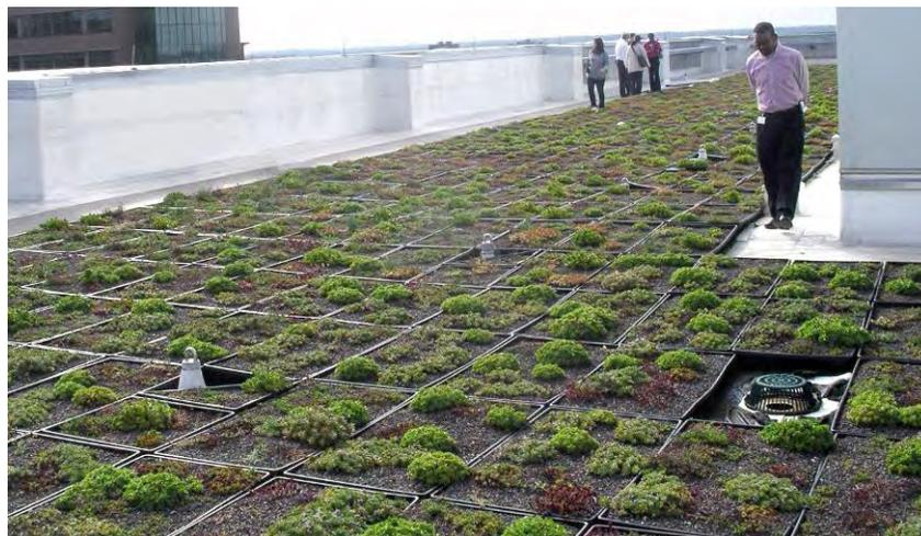
**Figure 4-15. Modular Green Roof System Installation**
