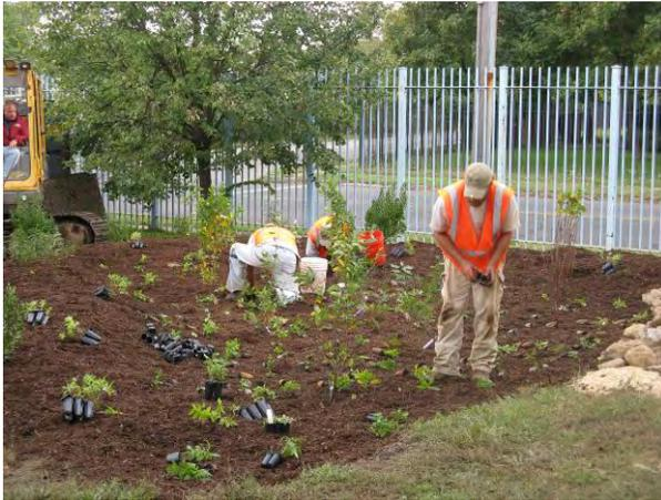
Stormwater retrofits are structural practices installed in upland areas to capture, treat, and store or infiltrate stormwater runoff before it is discharged to a water body or wetlands. Stormwater retrofits include end-of-pipe treatment measures installed in the downgradient portion of a storm drainage system to treat flows prior to discharge, as well as structural practices that can be added to existing, developed sites including LID and green infrastructure approaches.
