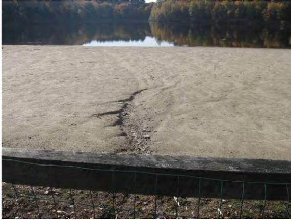
**Beach erosion resulting from stormwater runoff at Wolfe Park**
