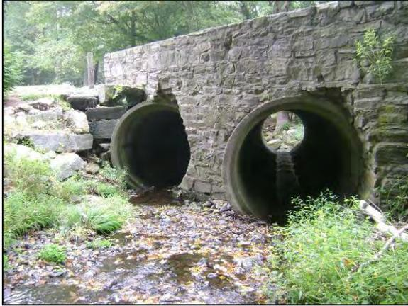
SC-01 is a twin 72-inch culvert for the stream crossing at Strobel Road, marking the beginning of the reach.
