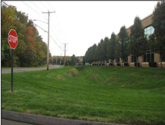
A large dry detention stormwater basin collects runoff from the site and provides water quality and quantity treatment.
