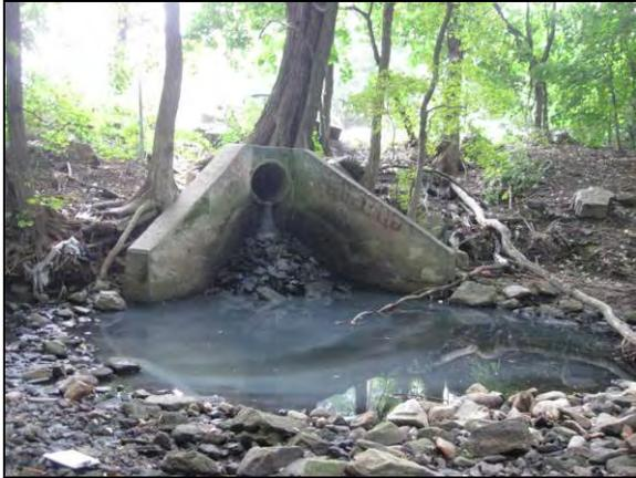
Dry-weather discharge at OT-02 was determined to be illegal connections of residential discharge.
