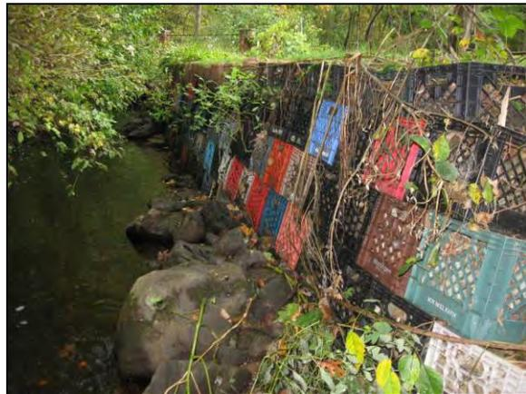
Retaining wall constructed of milk-crates filled with rocks and cement along UWB-03.
