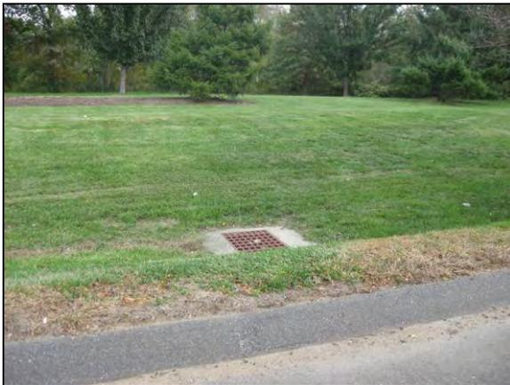
The catch basin is located in a grass swale to allow for infiltration prior to entering the storm drainage system.
