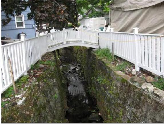
Stream channelization near the Chopsey Hill Road stream crossing disconnects the stream from the floodplain, increasing peak flow velocity.
