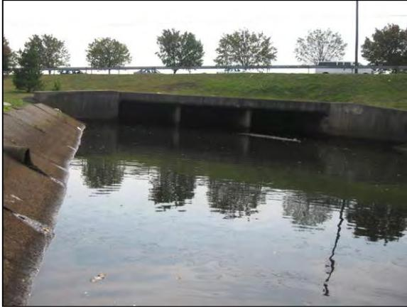
Reach LPR-05/06 is an underground culvert discharging at a triple box culvert in Beardsley Park.
