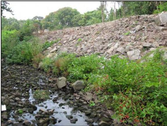
ISL-03B is channelized with rip-rap and placed stone in the stream channel.
