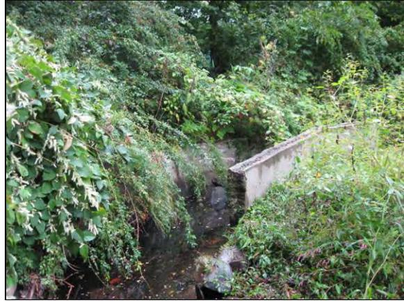
Retaining walls in this section of the reach are being actively undercut due to upstream development and lack of floodplain connection. Japanese Knotweed and other invasive species are prevalent in this area.
