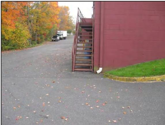
Downspouts discharge to impervious surfaces at Chuck's Corner Shopping Center.
