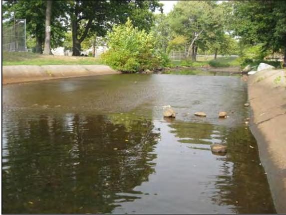
The construction of a fish apron across this concrete culverted section of the reach would allow fish passage during periods of low flow.
