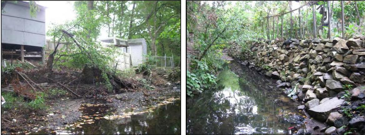
The biggest problem along reach ISL-04 is impacted buffers on residential properties. Many structures are built close to the stream bank (left) and a stone wall was constructed as a retaining wall to the river (river). Buffer encroachment prevents adequate connection to the floodplain.
