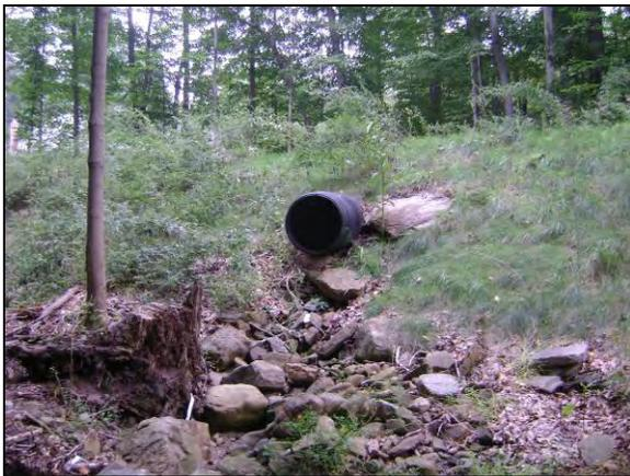
Tributary outfall OT-01 has an approximately 3-foot drop to the channel which is causing erosion and scour around the outfall.
