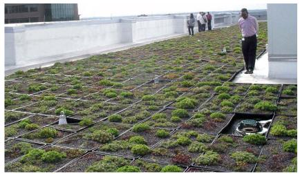
Figure 4-9. Modular Green Roof System Installation
