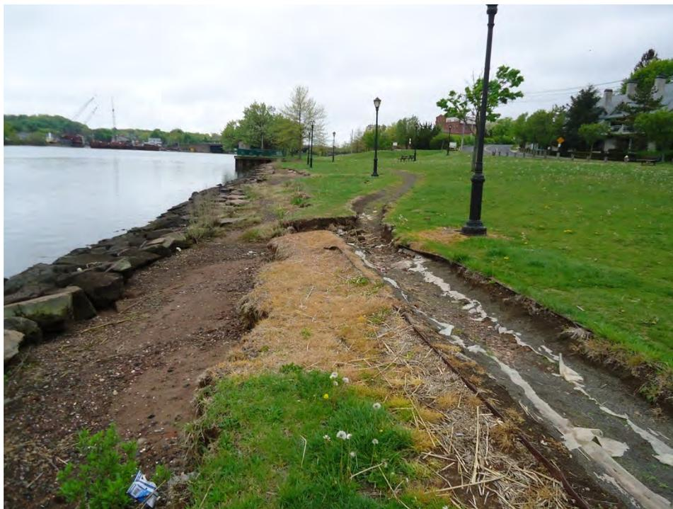
**Figure 2.1.1. Shoreline Erosions and Erosion on Walkways at Quinnipiac River Park**
