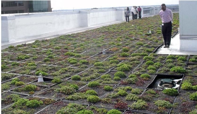
**Figure 4-6. Modular Green Roof System Installation**
