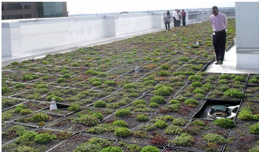
**Figure 5. Modular Green Roof System Installation**
