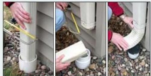
Disconnecting your downspout is a simple and effective way of reducing stormwater runoff. (Photo from [grandbuilding.ca](http://grandbuilding.ca))
