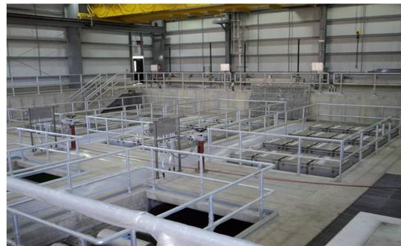
MDC Hartford: Recently completed final treatment process (disinfection using ultraviolet light)
