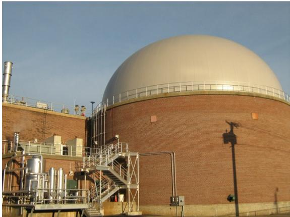
Norwich WPCF: Energy recovery project, utilizing waste gases from the treatment plant to generate electrical power
