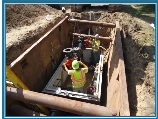
Bolton Lakes: Installation of low pressure sanitary sewers as part of the small community project to protect the Bolton Lakes. (Photo courtesy of Fuss & O'Neill, Inc.)
