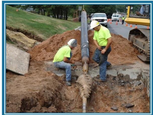
Bolton Lakes: Directional drilling to install pipe with minimal disturbance to surface features (such as State Route 44) (Photo courtesy of Fuss & O'Neill, Inc.)
