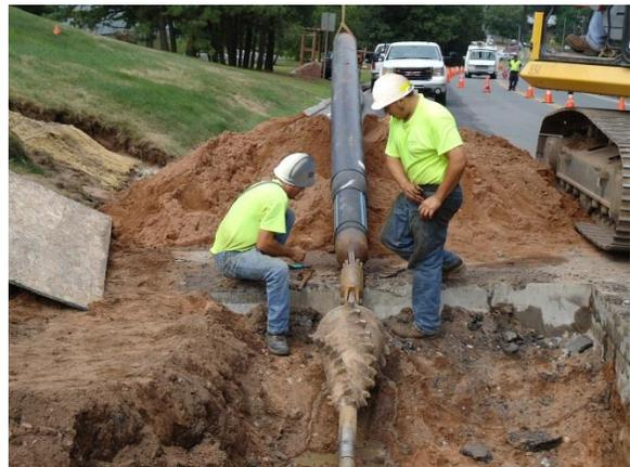
Bolton Lakes: Directional drilling to install pipe with minimal disturbance to surface features (such as State Route 44)
