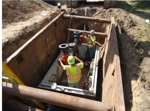
Bolton Lakes: Installation of low pressure sanitary sewers as part of the small community project to protect the Bolton Lakes.
