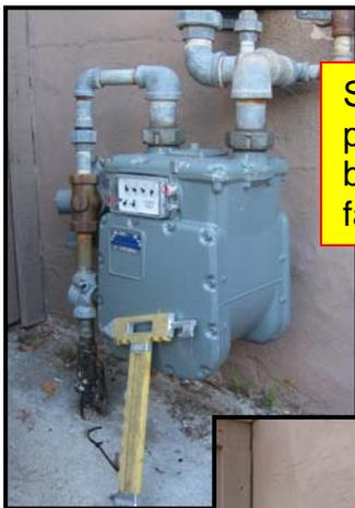
Shut off gas at meter to prevent gas leak from broken gas line at the facility
