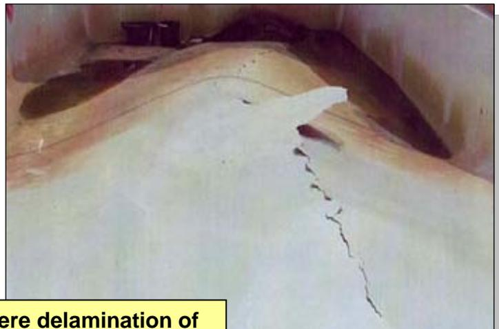
**Severe delamination of fiberglass pool surface.**
