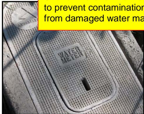
Shut off water at the main to prevent contamination from damaged water main
