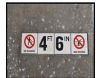
**DEPTH MARKING LINES** are only required for pools that have a maximum depth greater than 5 feet. It must be a 4 inch wide straight line of contrasting color across the bottom of the pool at the 4 ½ foot depth marker. If the pool is greater than 5 feet deep and also has a break-in-slope, it is required to provide both a depth marking line and float line with buoys.
