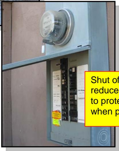
Shut off electricity at main circuit box to reduce risk of fire or electrical shock and to protect equipment from power surge when power is restored
