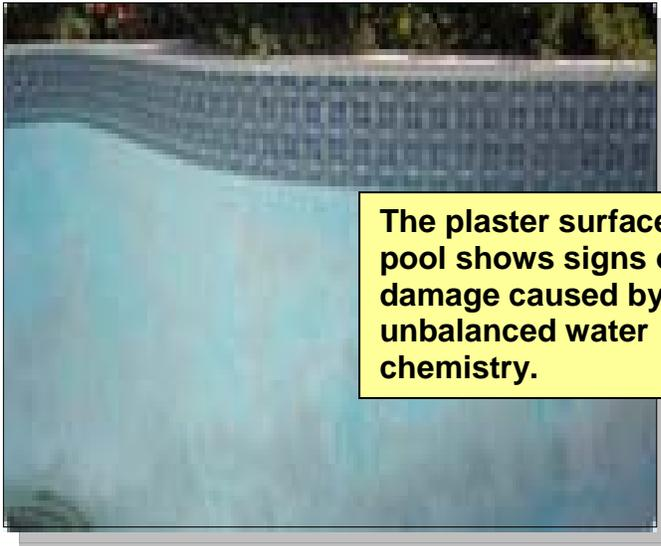
**The plaster surface of this pool shows signs of damage caused by unbalanced water chemistry.**
