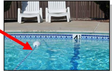
**DEPTH MARKERS** are required for all pools and spas and must be located at each end of the pool and at the deepest and shallowest depth of the pool.
